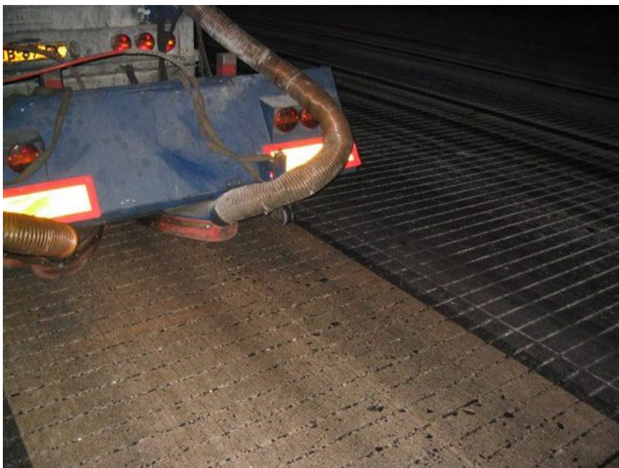
FIGURE 16: RUBBER REMOVAL CONCRETE
