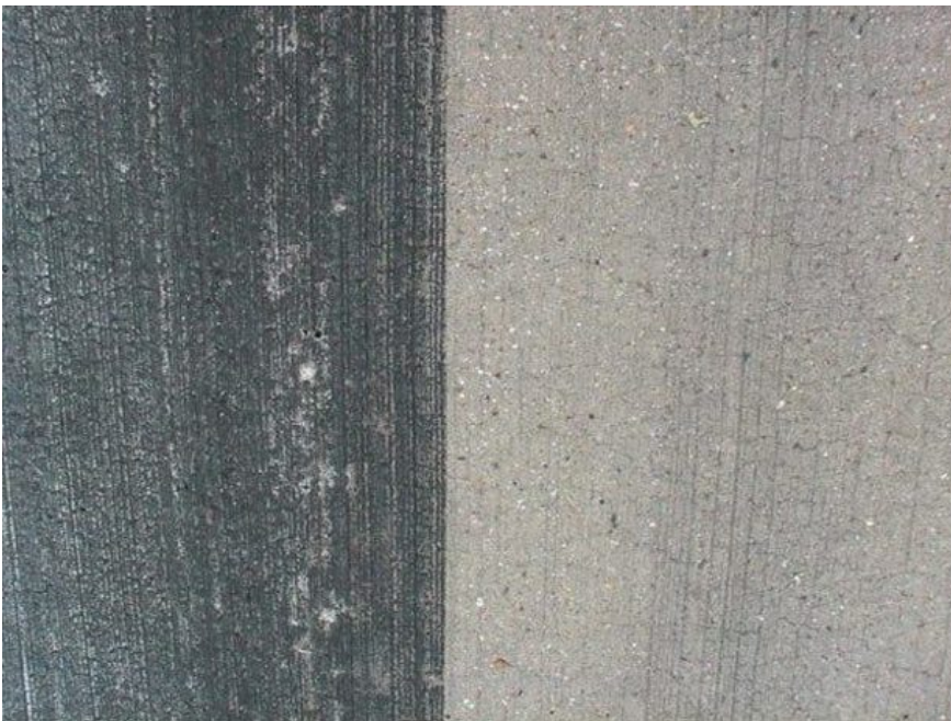
FIGURE 12: CONCRETE RUBBER REMOVAL
