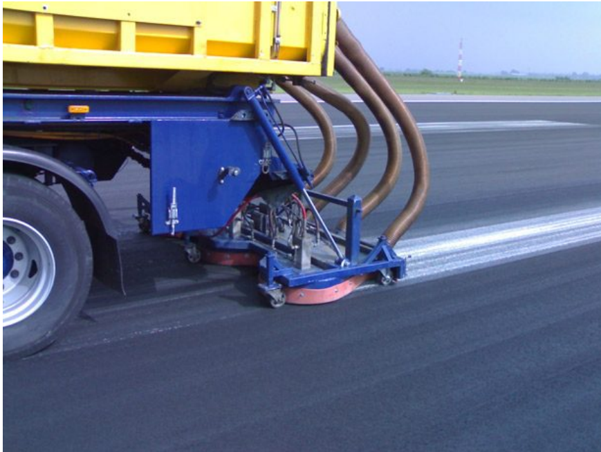
FIGURE 15: CLEANING RUNWAY LINE MARKINGS
