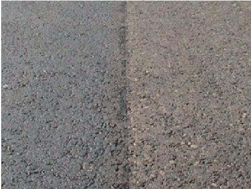
FIGURE 13: ASPHALT RUBBER REMOVAL
