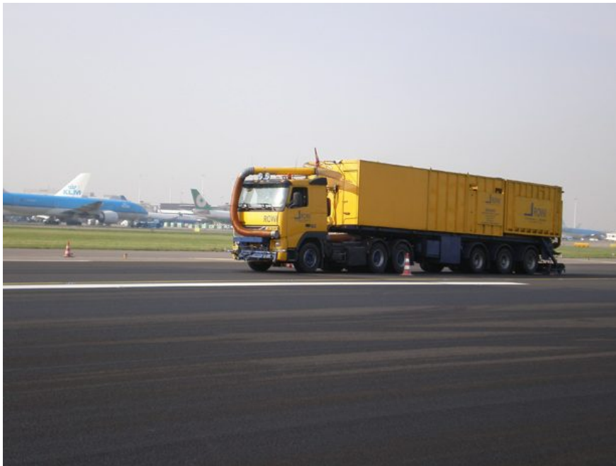
FIGURE 10: HIGH PRESSURE RUNWAY CLEANING
